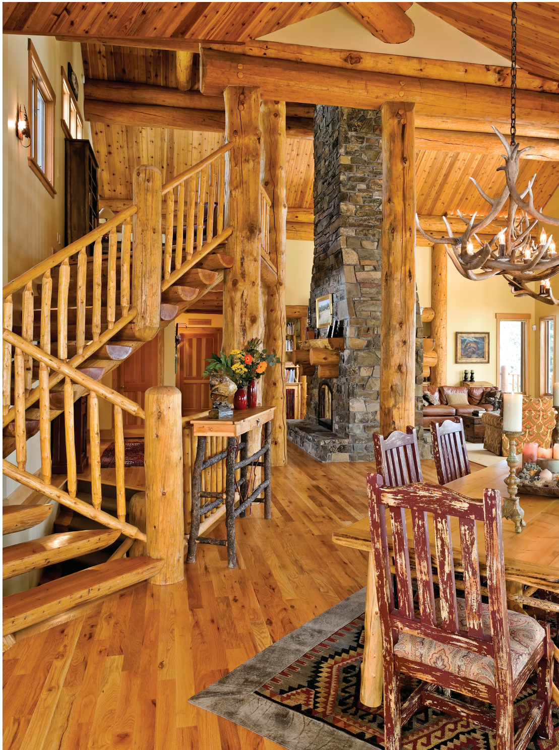
Even the spacious great room has a cozy, intimate feel. This Big Sky lodge incorporates conventional frame construction with load bearing log post-and-beam features.
